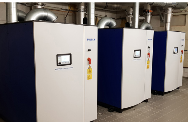
The new installation of three HST 20 units
