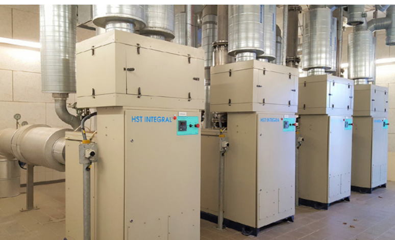
The original installation of four turbocompressors
